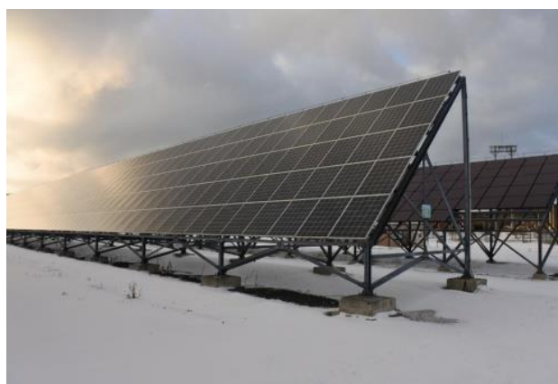
(Wakkanai Solar Power Plant)
